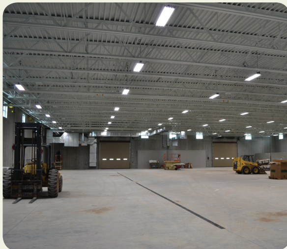
Plymouth Utilities' 24,900 square-foot garage facility. The garage can hold up to 30 vehicles and will be heated with a geothermal in-floor radiant heating system and lit with Orion's energy-efficient 32-watt, T8 motion sensor equipped light fixtures.
